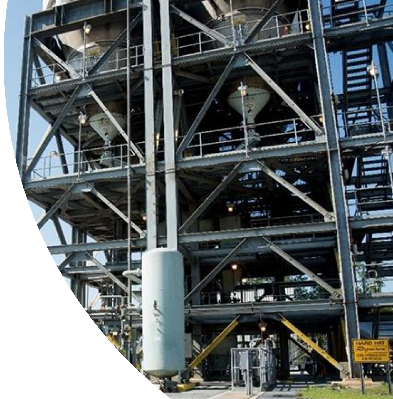
Saltstone Grout Facility at Savannah River
