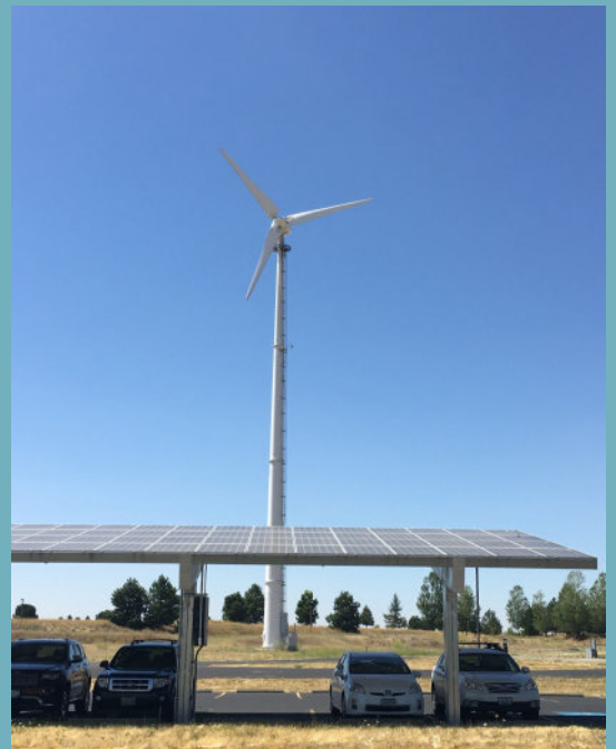
Wind turbine and solar array at the Tamástslíkt Cultural Institute
