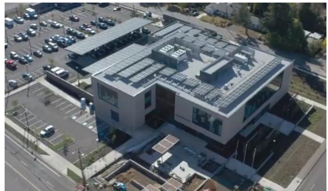
The Beaverton Public Safety Center has a backup power system that includes a generator, solar energy, and a battery energy storage system.
