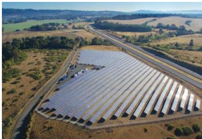
This nearly 3-MW solar array outside Willamina launched Portland General Electric's Green Future Solar Program in 2016. PGE customers could "buy" 1-kW blocks of solar.
