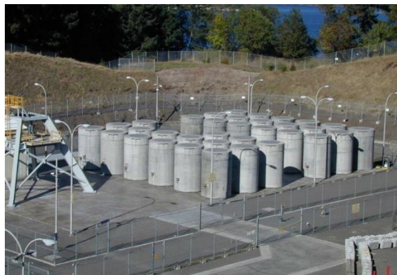
Trojan Nuclear Plant spent fuel casks.
