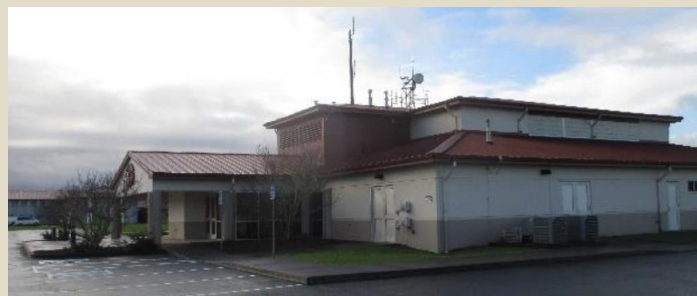
Emergency Operations Center, Building 7022
